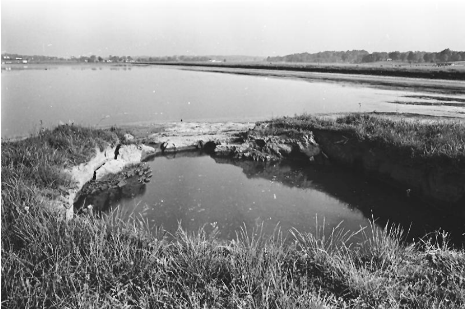
In the foreground of this May 15, 1978, photo is the small sinkhole that formed in the peninsula within the city's lagoon. (Photo courtesy West Plains Daily Quill)
