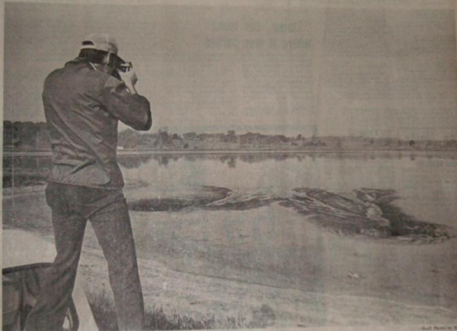
MORE SEWAGE GOES UNDERGROUND —Dr. Pat Phillips, state epidemiologist, from Poplar Bluff, photographed a second collapse in the floor of the West Plains sewage lagoon that occurred overnight, causing an estimated amount of the remaining sewage to drain into underground caverns. The city began draining as much of lagoon's contents into another nearby cell when the second break was discovered late Tuesday. The first break on May 3 appeared to seal itself after the initial loss of 90th volume gallons. The hole on the left was about six feet in diameter. The hole on the right was about eight feet across and sewage was taken about 1 1/2 in. holes. Both were 6' larger in the cells contained sewage from the collapsed cell. The hole on the left was the problem mentioned in the May 3 leak occurred.
